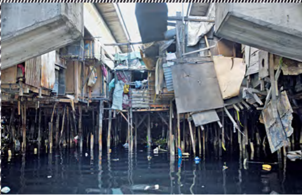
AN ILLEGAL SETTLEMENT MADE OF BAMBOO, CARDBOARD AND PLYWOOD IN THE PHILIPPINE CAPITAL.
