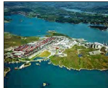
Metal plant, Karmøy, Norway
