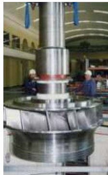
Hydro electric powerstation, Rjukan, Norway:
