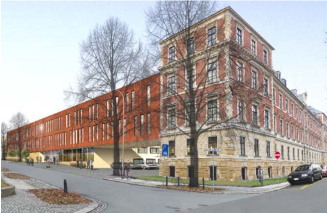
Justice Centre, Chemnitz Completion: December 2008 Operation over 20 years, without equity commitment
